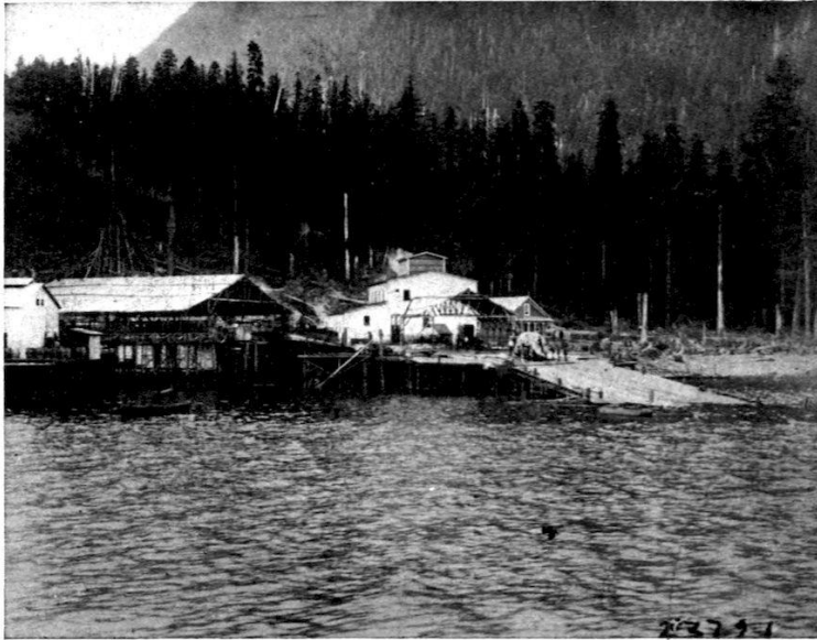
A modern shore whaling station at Kyuquot, Vancouver Island, B. C. The flensing slip, carcass platform and wharf are shown in the foreground. In the background is the manager's dwelling.
