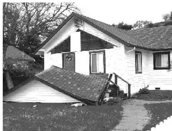
Figure 6 - San Simeon Earthquake, Dec. 22, 2003 The collapsed porch was not adequately attached to this single-family residence.
