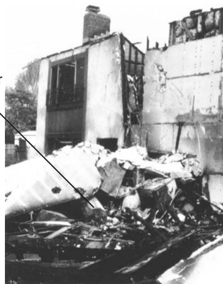
Figure 7 - The unbraced water heater in this home fell during an earthquake; the resulting fire destroyed the home.
