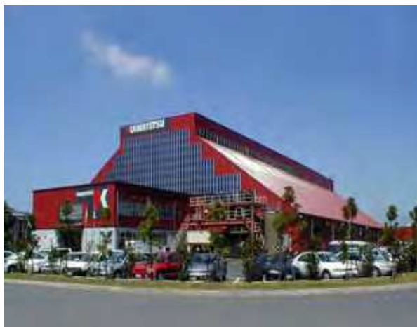
Photo 2. MSW gasification plant in Chiba (Japan)
