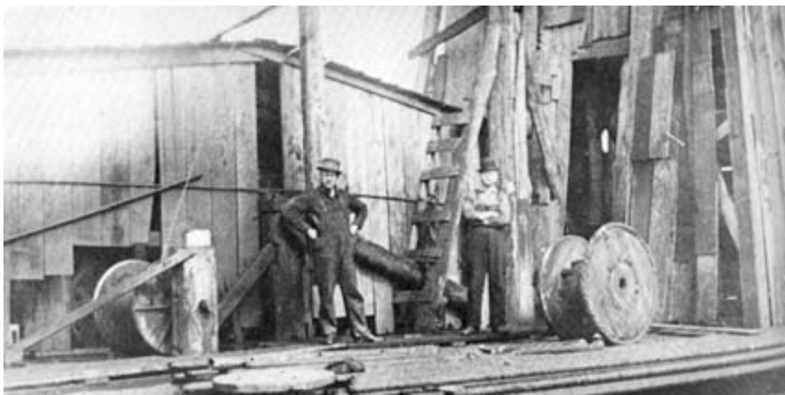
Below: This structure was typical of the cable tool drilling rigs that sprung up all across Oklahoma oil fields in the early 20th century. This rig, built from nearby timber, stood during the boom at Red Fork.
