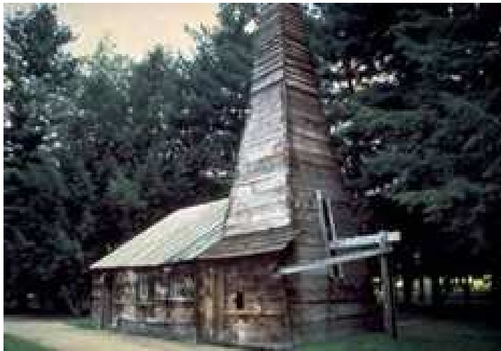
Fig. 1. A Reconstruction of 'Colonel' Drake's First Well in Titusville, Pa (Source: API)
