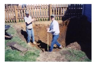
Keep in mind that you want to keep the top 'shoreline" edges pretty level. The reason for this is that once you put the liner in and fill the pond with water you won't have a large piece of the liner showing
