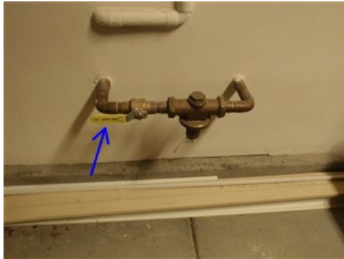
Main Water Valve at Pressure Regulator
