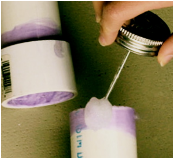
Solvent welding a PVC fitting
